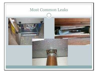
Photo 1 – Furnace cabinet (for multiple position cabinets there is a removable plate - that plate is not sealed)
